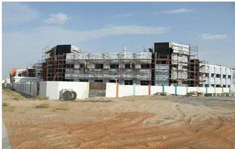
Project : Al Zayediya school Al ain
