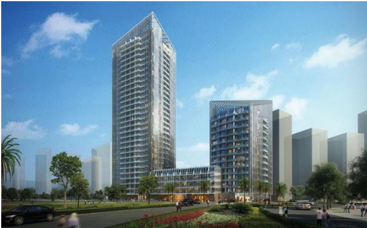
Sparkle Tower, 3B+G+14/29 Twin Tower at Marsa, Dubai, UAE
