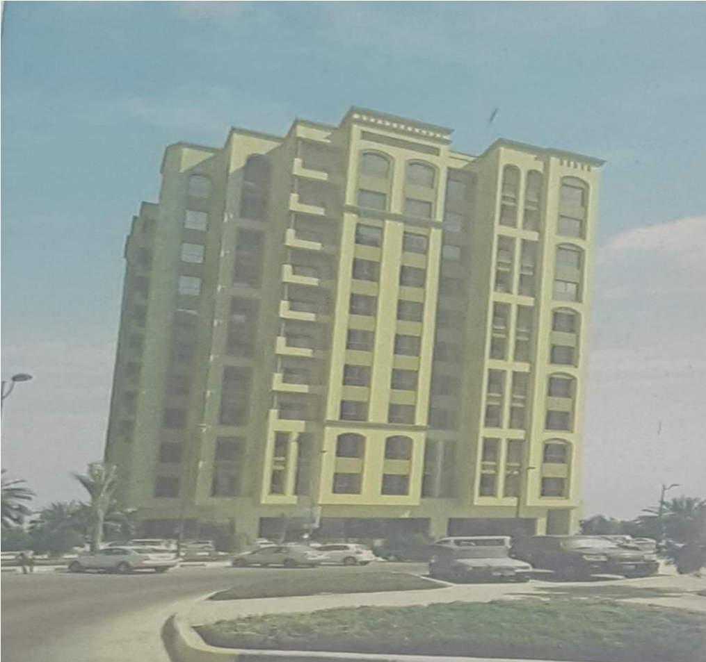
2B+G+10F Residential Building, Al Barsha 1
