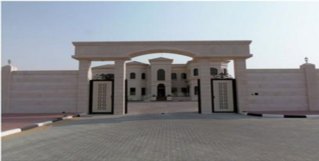
Project : Shaikh Palace, Ajman
