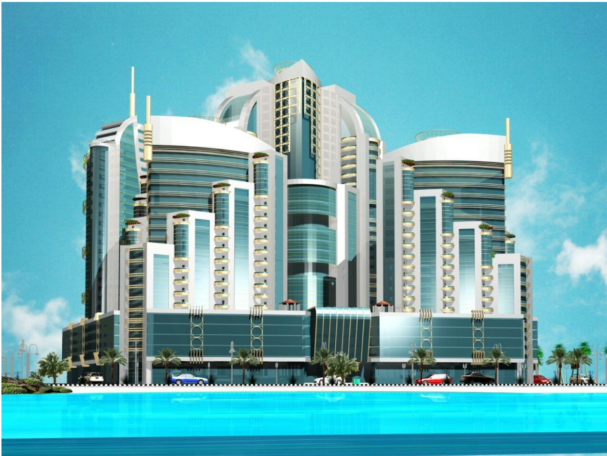
Orient Tower (G+3P+25 F 4 ,Towers) Al Bustan, Ajman, UAE
