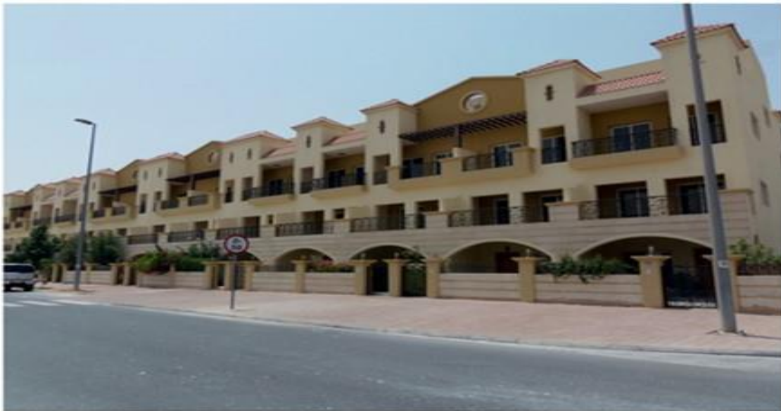
Project : Jumaira village 2 Dubai
