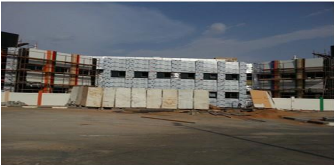
Project : Hessa Bint Mohamed School, AL Ain
