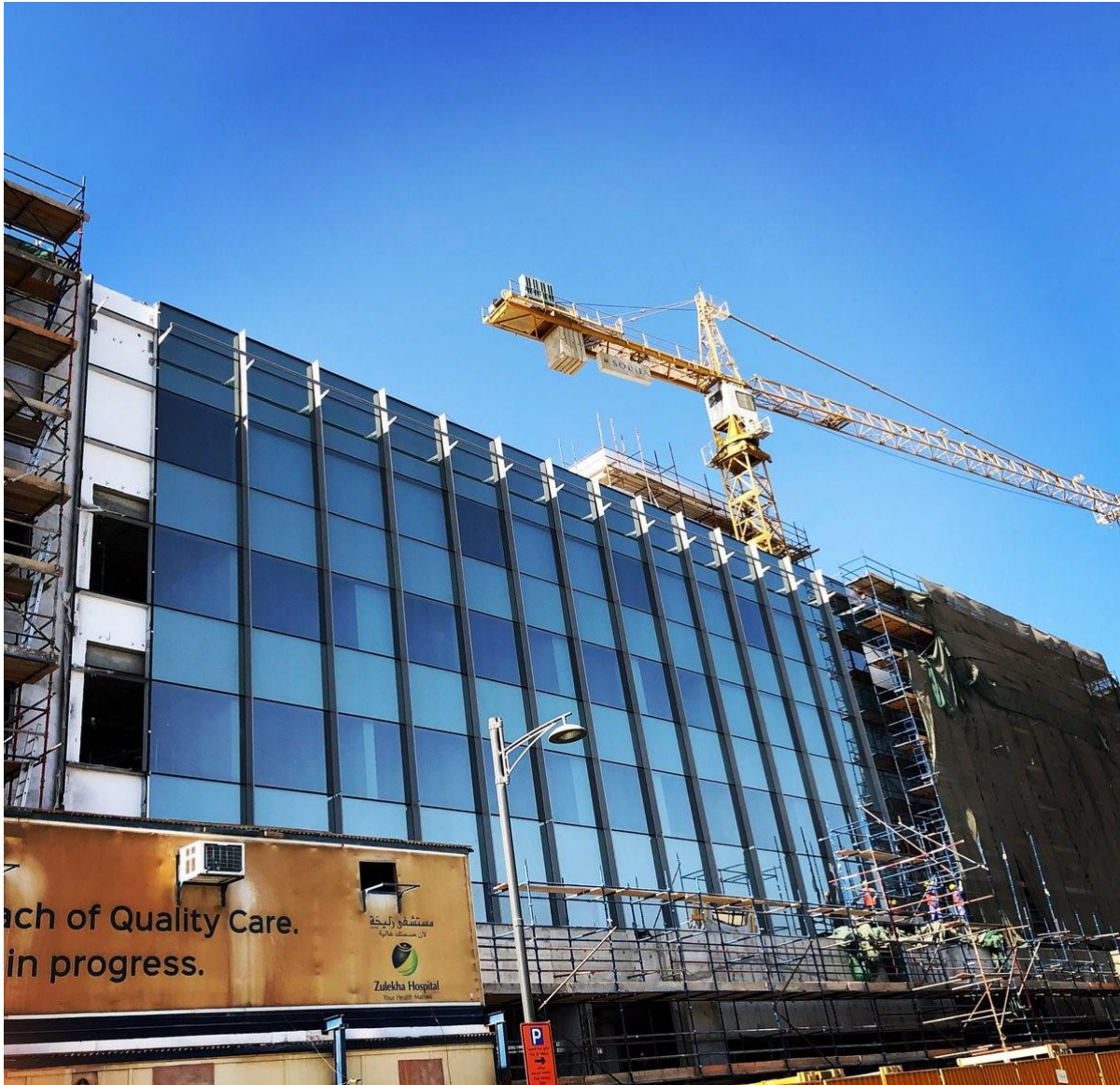
Zulekha Hospital, 3B+G+4 Hospital Building, Al Nahda, Dubai, UAE
