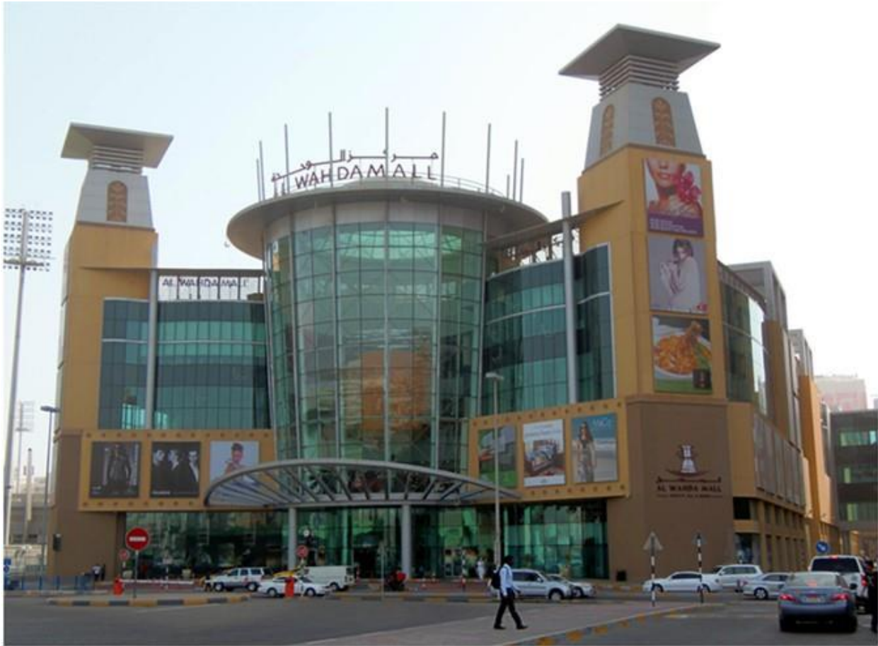
Project : Wahda Mall Abu Dhabi
